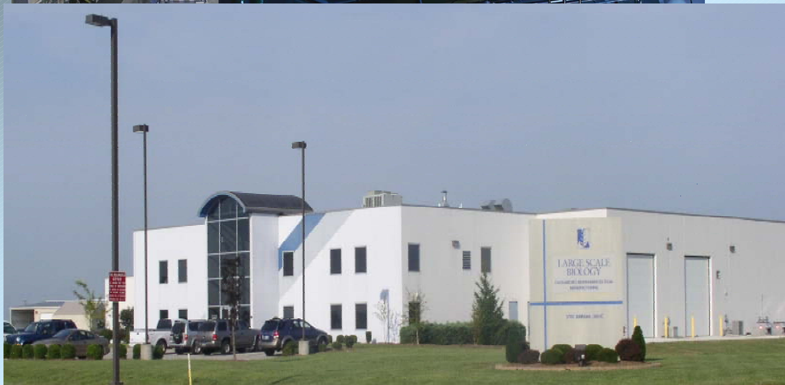
Large Scale Biology - Plant- Made Biopharmaceutical Facility Owensboro, Kentucky
